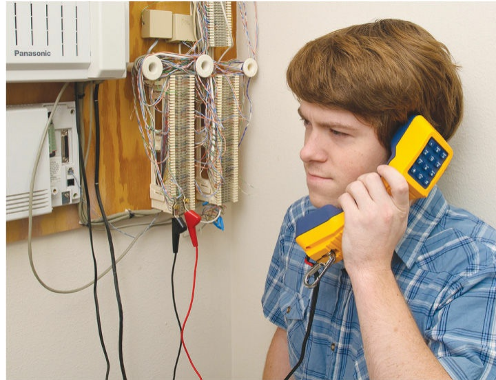
Figure 5-69 Technician with a butt set
