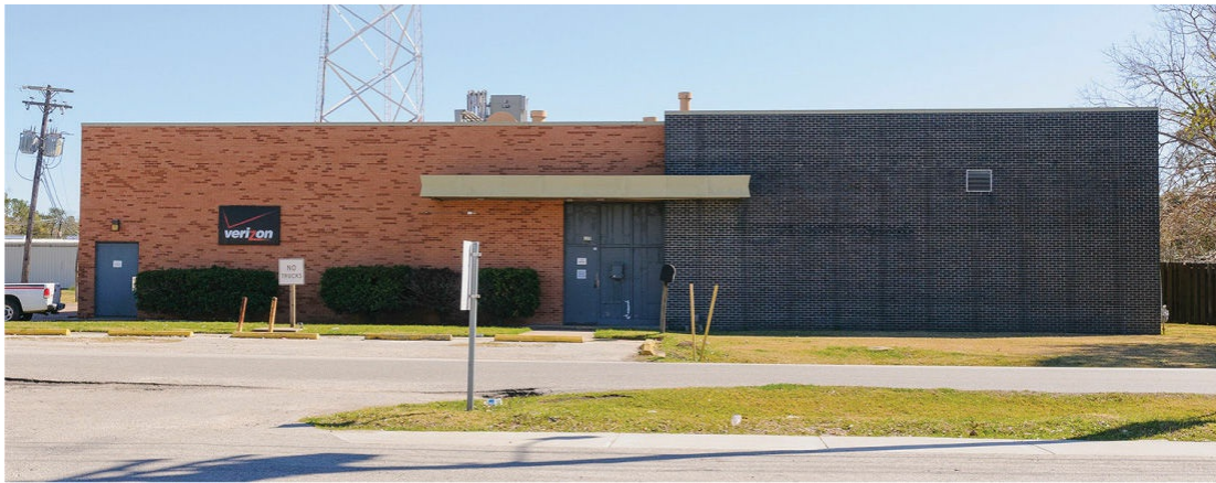
Figure 13-6 A central office building
