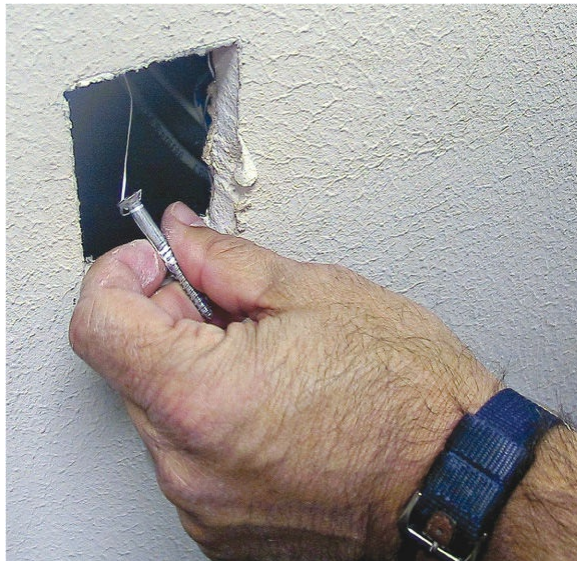
Figure 5-33 Locating a dropped pull rope
